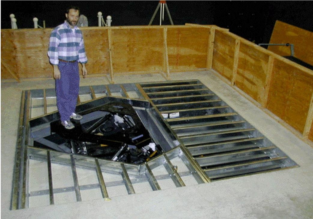
Figure 4. CAVE floor substructure and motion base under construction, February 13, 2001.
